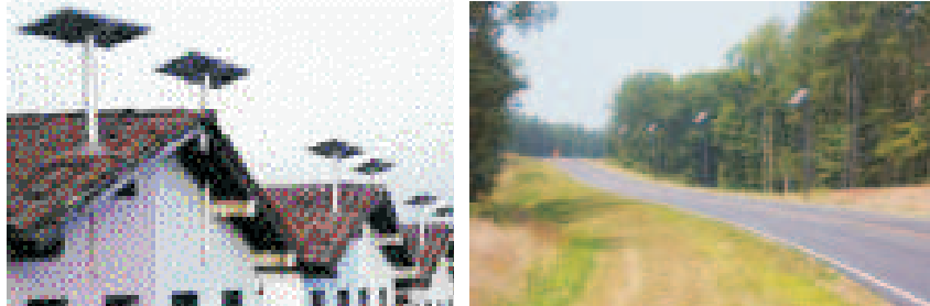
Figure 12.5 Photovoltaic Domestic and Streetlights
