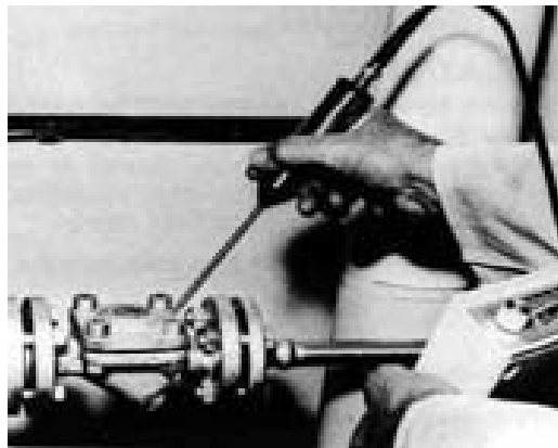
Figure 3.16 Ultrasonic Testing
