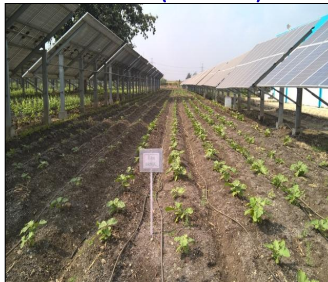
2x1 MW Distributed Solar Power cum Agriculture Pilot Projects -2016
