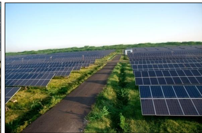
5 MW Solar Plant at SLPP
