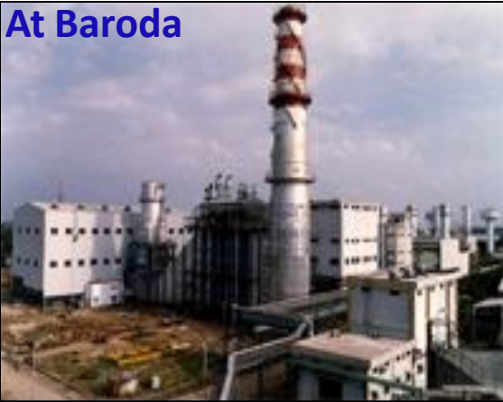
Gas Based Power Plant
